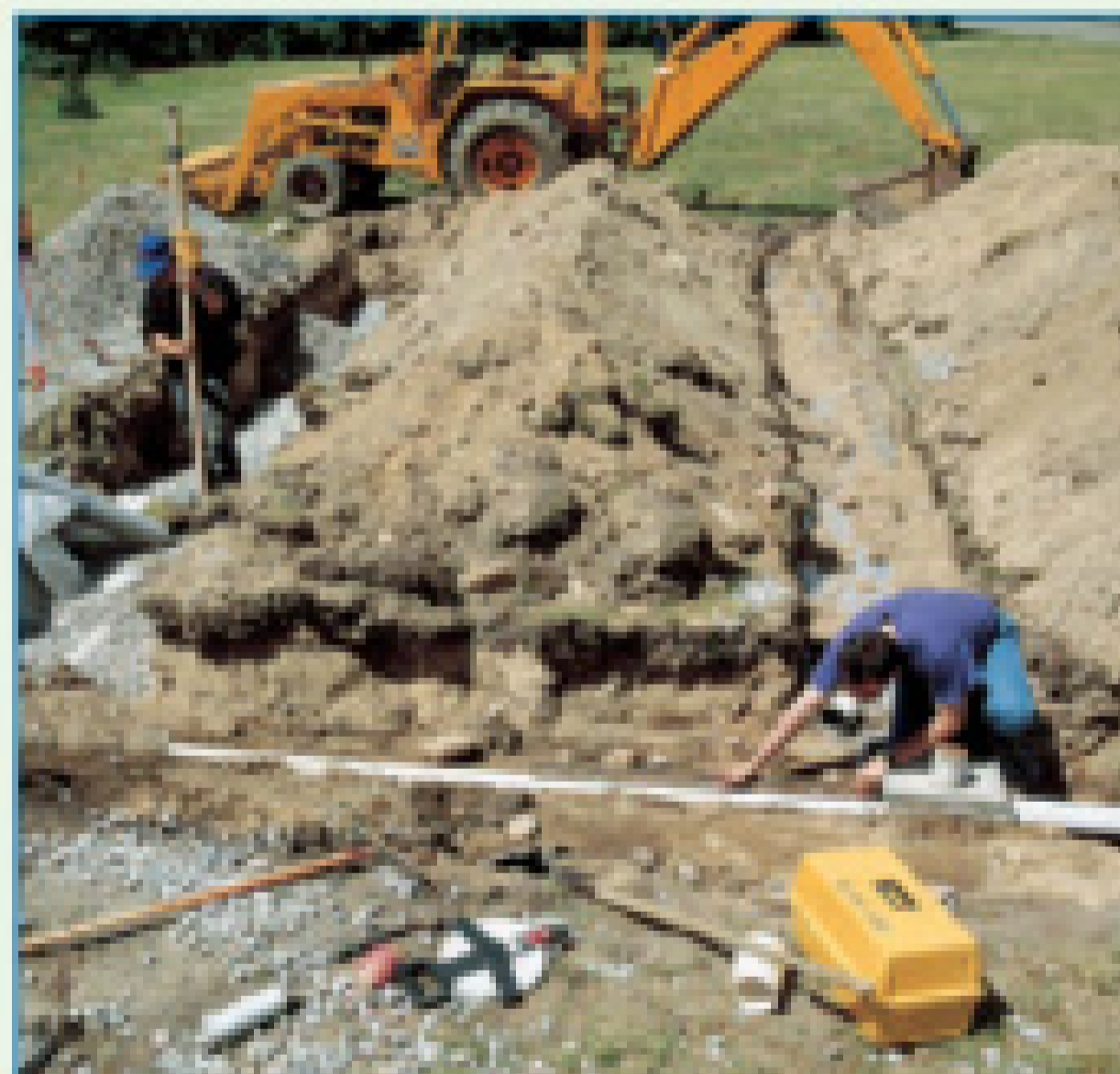
Typical Septic System Replacement Installation
