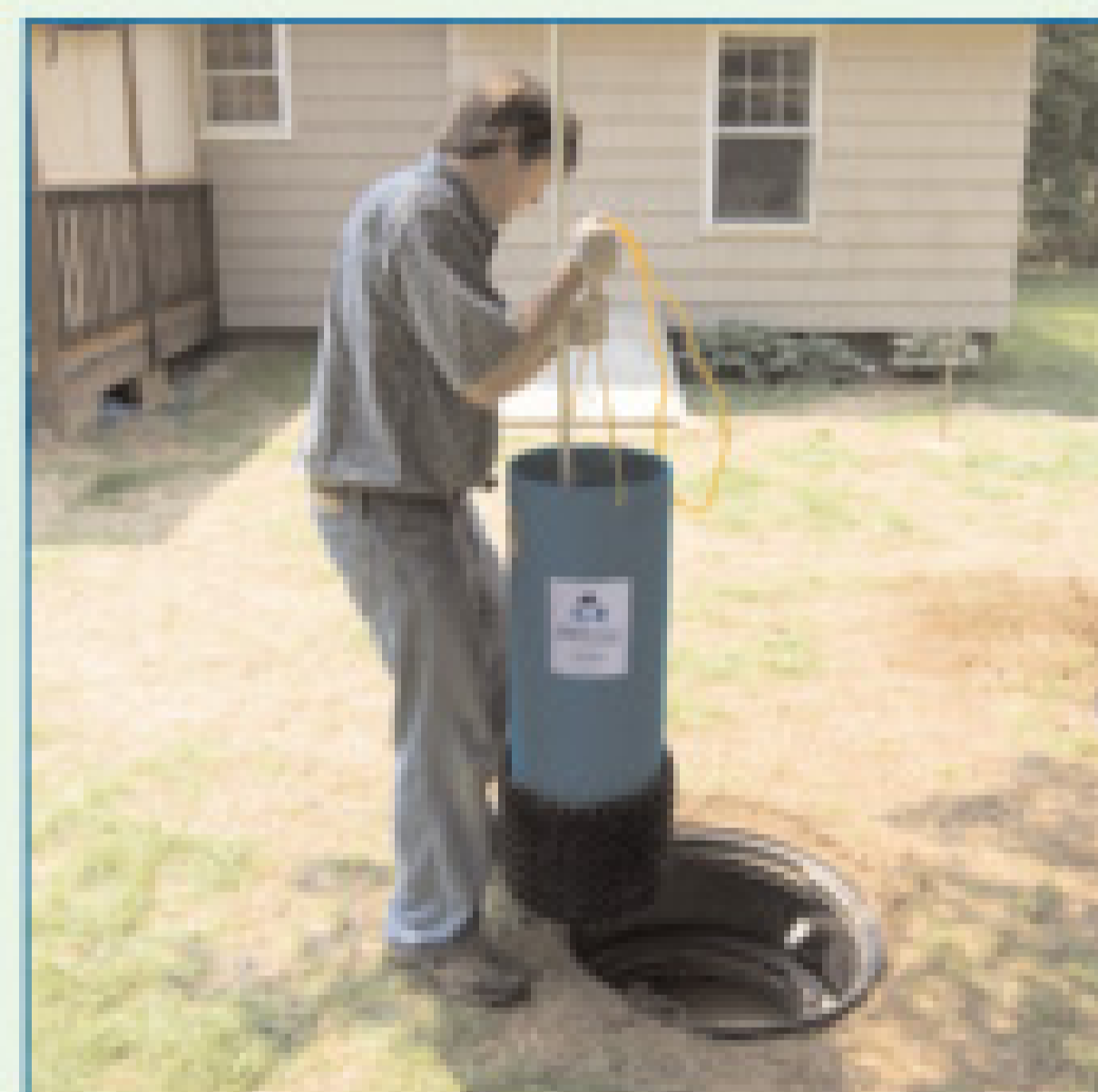
Aquaworx Remediator Installation
