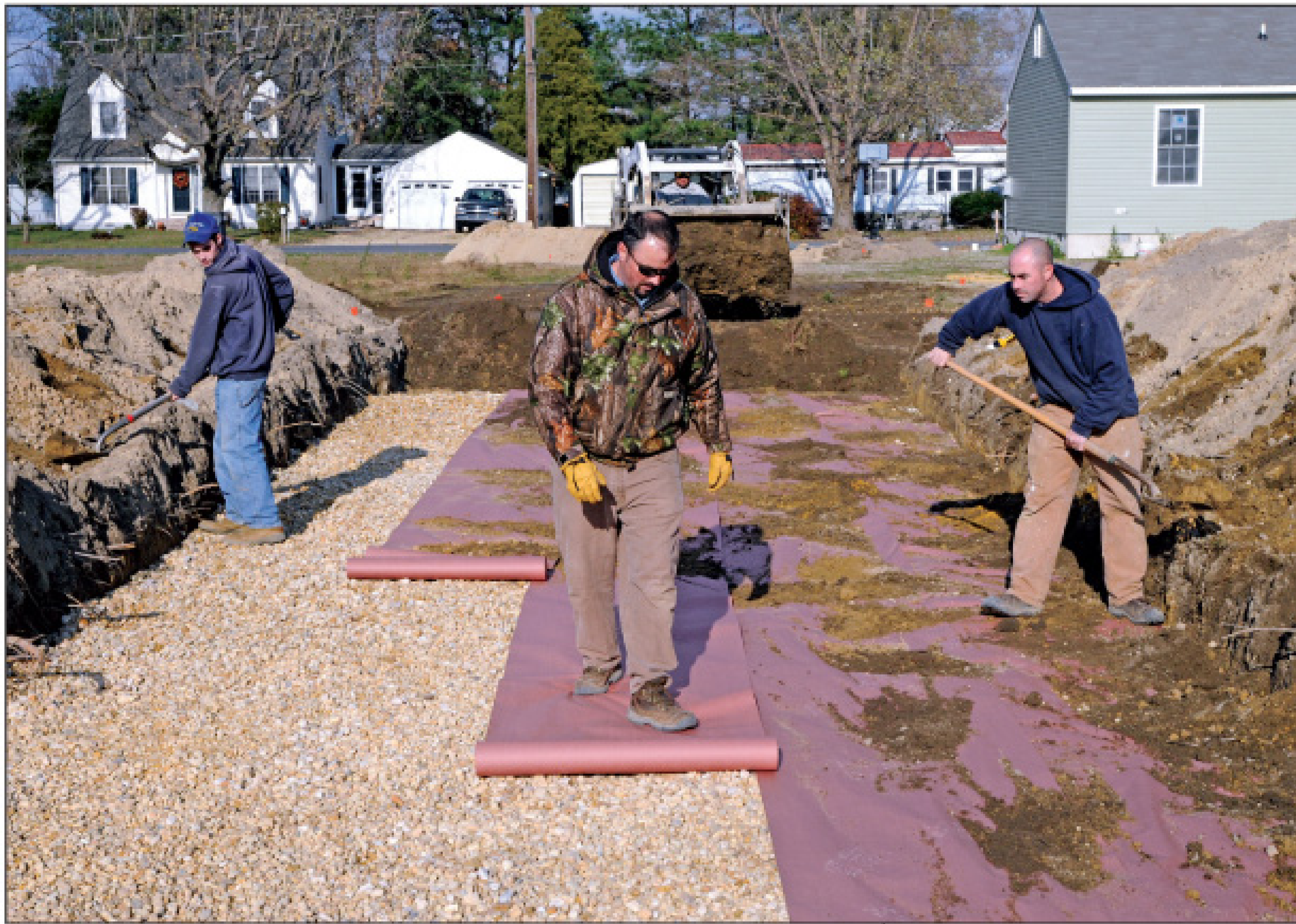
From left, Jeff James, Mike White and John Webb of C. White & Sons cover a drainfield with synthetic fabric and soil.
