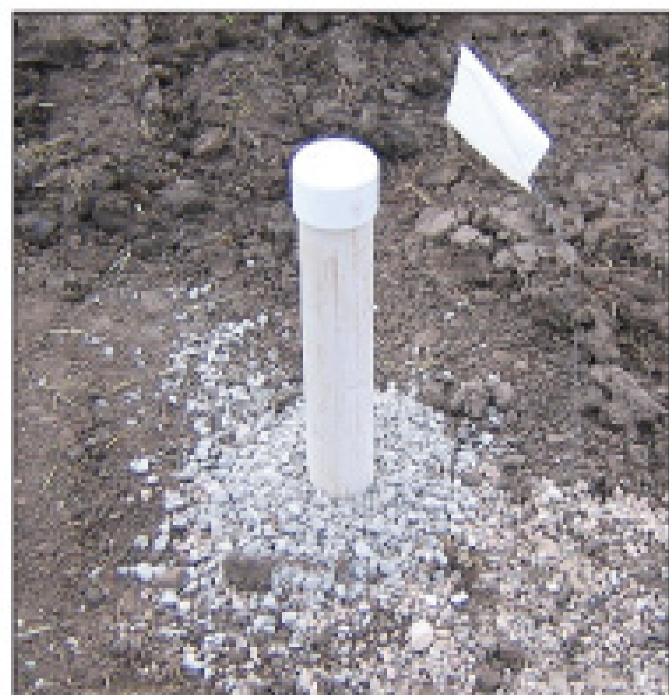
One of two PVC monitoring tubes near each end of the mound.
