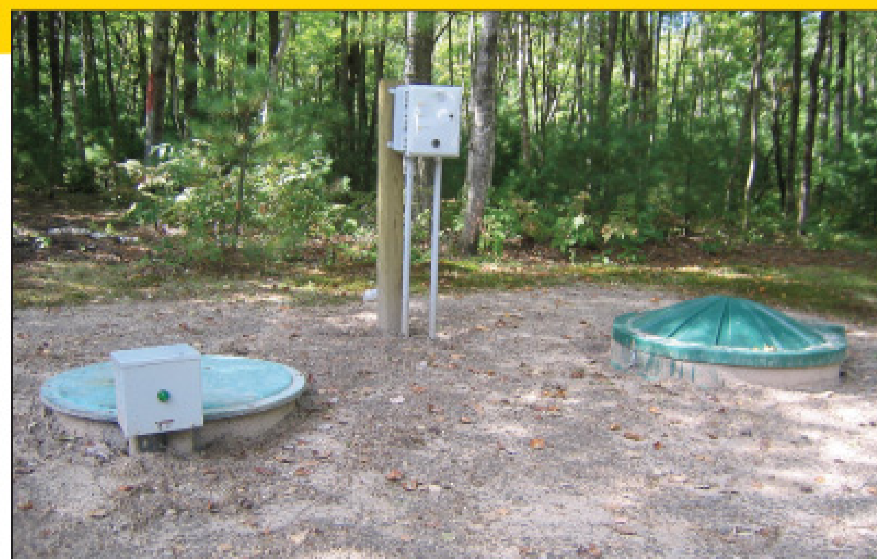
Above, the Multi-Flo aerobic treatment unit is to the right, the MF-080D4BR control panel is in the middle, and the pump chamber is to the left. Below, a shut-off device being installed. (Photos courtesy of Halverson Plumbing)
