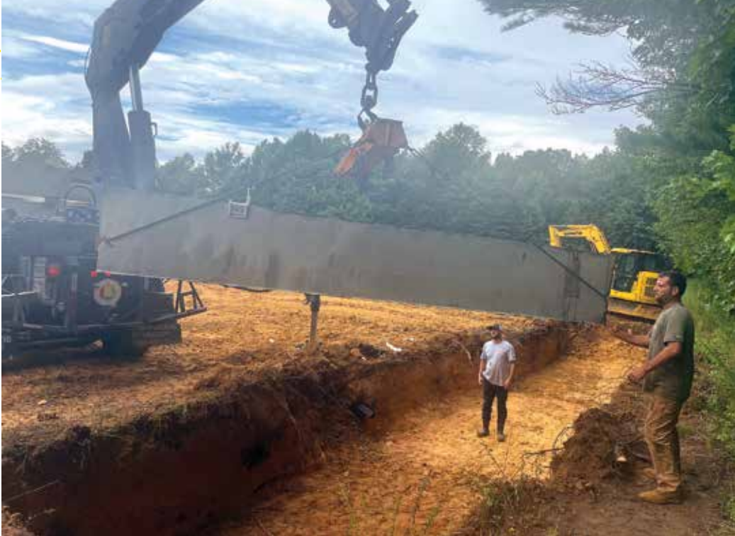
◀ Technicians set tanks for the Skyline School system in Scottsboro, Alabama.
