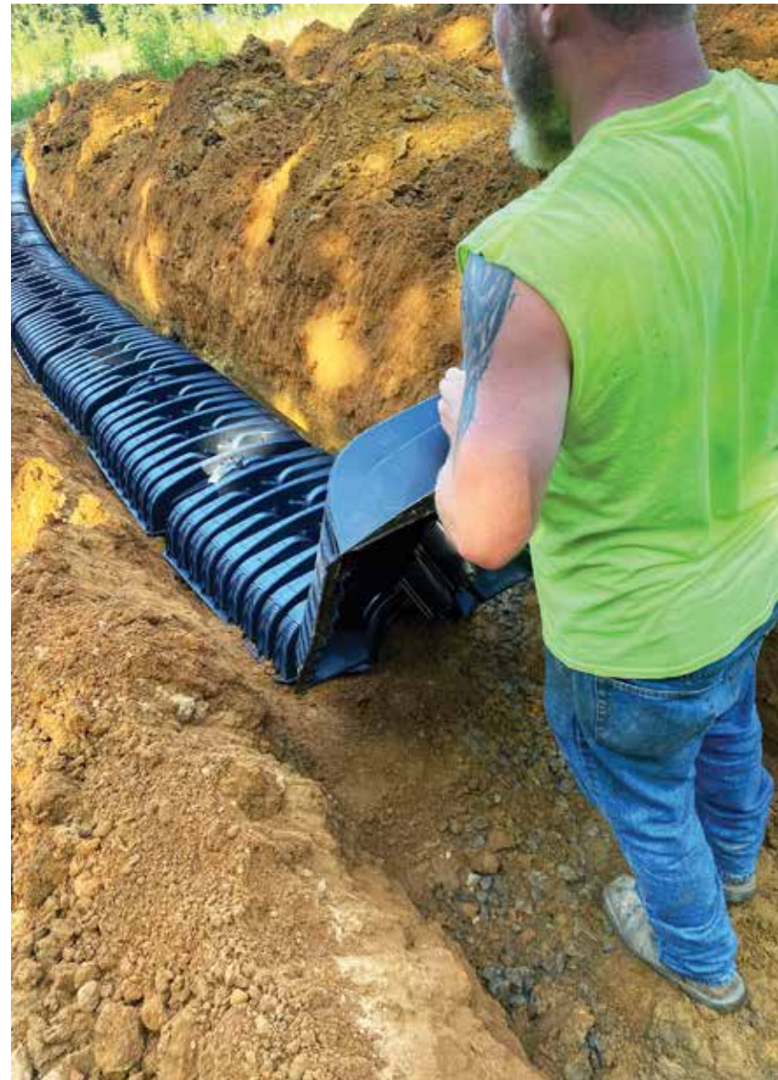
▼ A technician lays a row of Infiltrator chambers for the Skyline School system in Alabama. The system required 1,320 linear feet of chambers.
